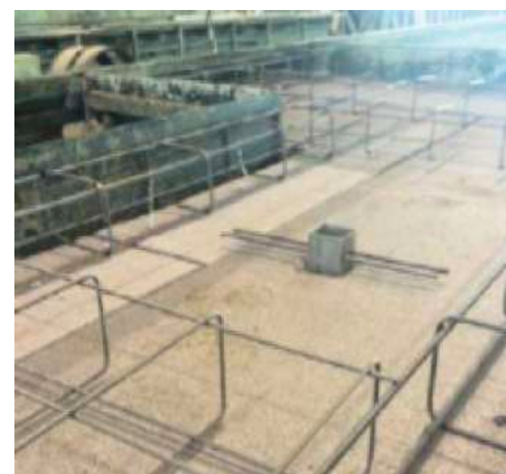
Isolante posato Insulation installed
