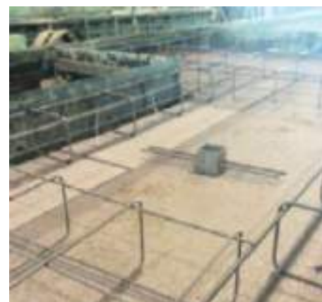
Isolante posato Insulation installed
