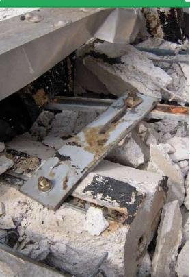
Collection of anchor channel systems as steel scraps, destined entirely for recycling.
