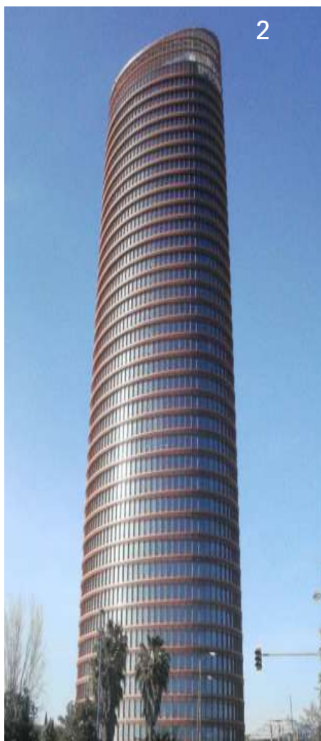
2 Torre Cajasol - Sevilla - Spain 5 Banca UBS - Bellinzona - Switzerland
